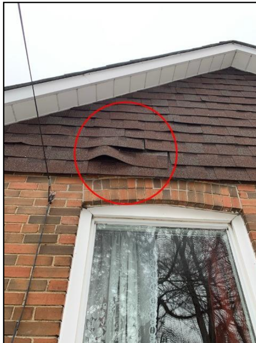
10. Loose, missing or torn tabs
