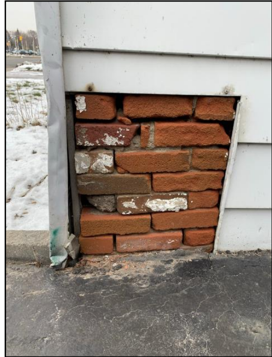
9. Mortar deterioration
