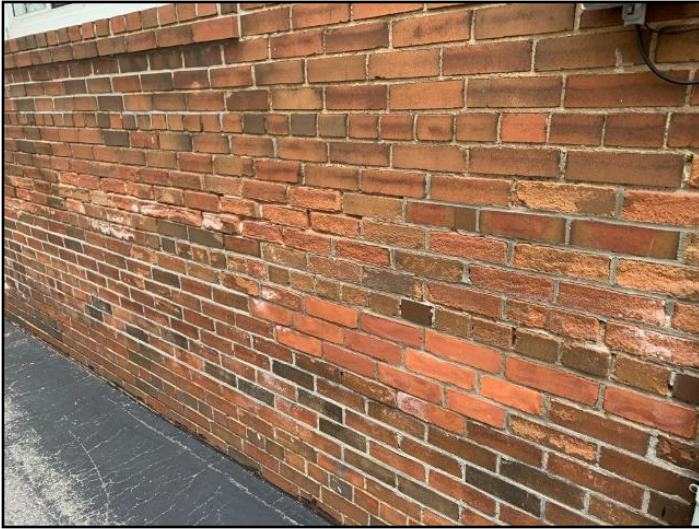
8. Mortar deterioration
